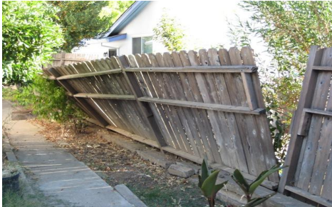
Documentation of property condition with digital photos, emailed or uploaded onto your online platform
